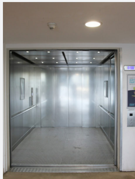
LARGE GOODS LIFT
